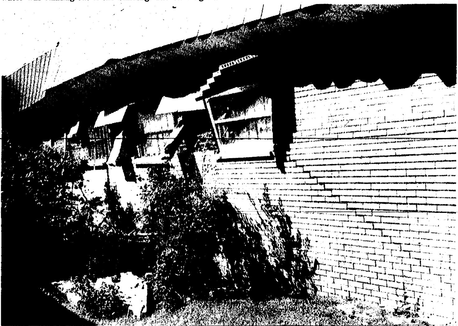
EXTERIOR WALLS of the Gregory Post Office buckled outward under the weight of a collapsed roof last Wednesday night or Thursday morning. The building had not been inspected as of press time but workers suspect accumulated water on the roof caused the cave-in.
